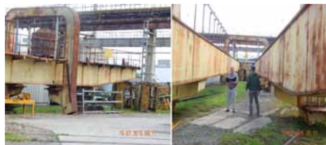
Figure 3. General view of the crane girders.
